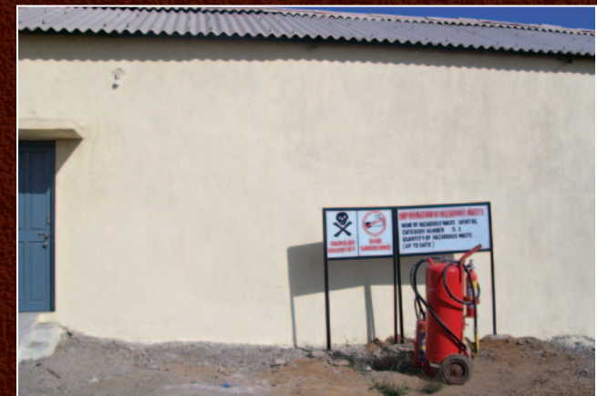
Hazardous waste storage facility at ATPS
