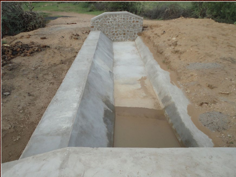
Wast weir of Chiyad pond, Nakhatrana, Kachchh
