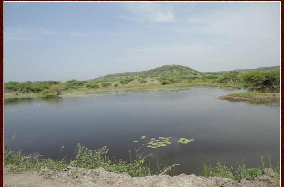
Checkdam at Khanot
