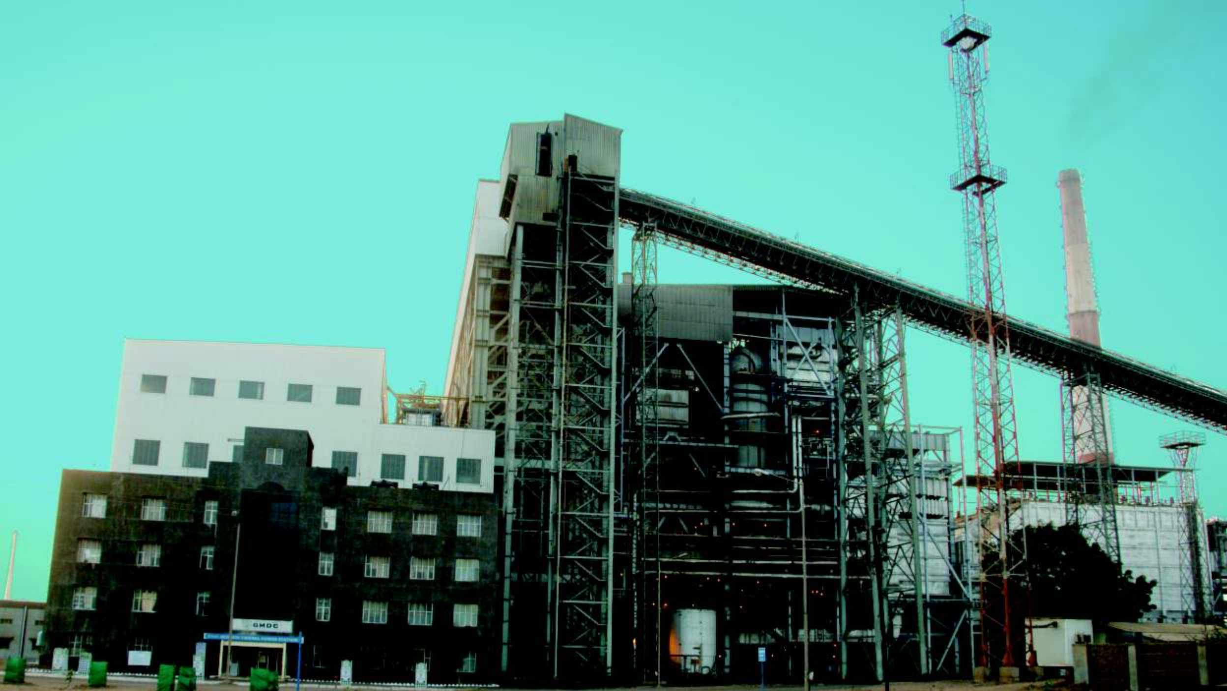
GMDC 250 MW POWER PLANT. CHHER
