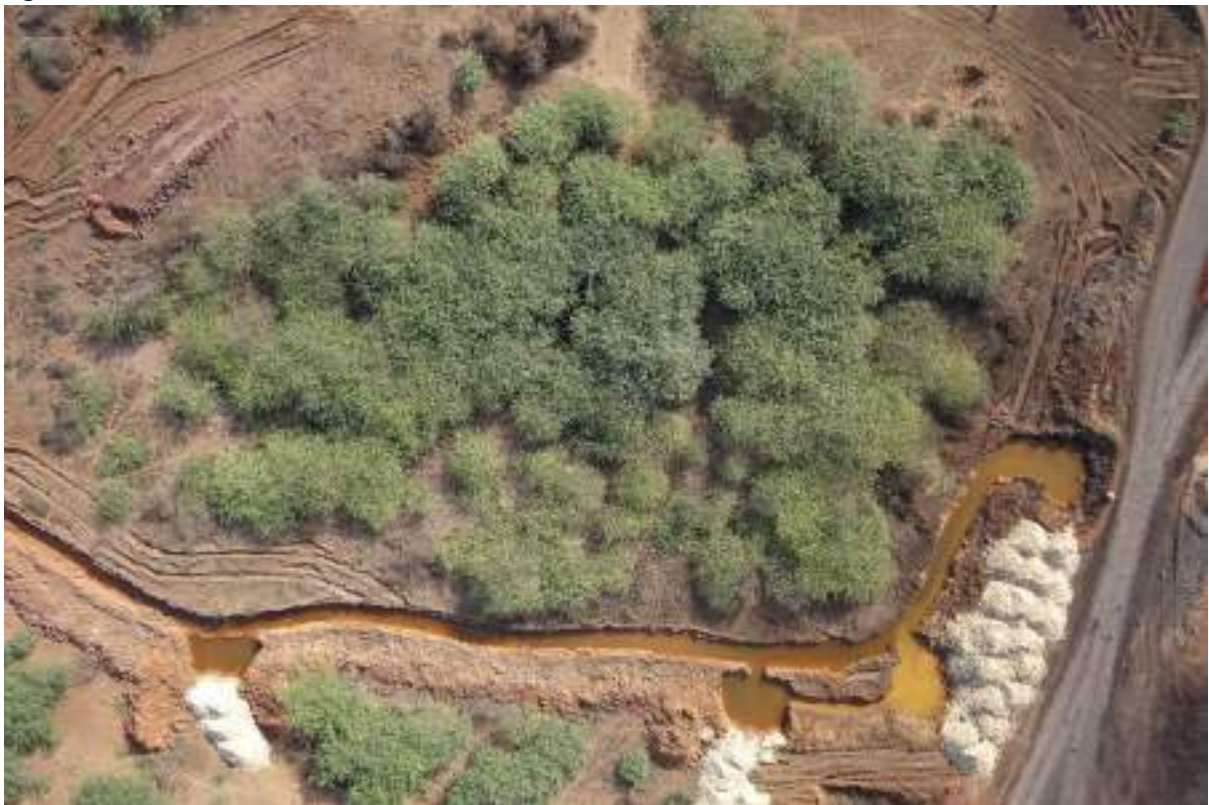
Fig 3.3.13 Aerial view of shrubs and drainage
