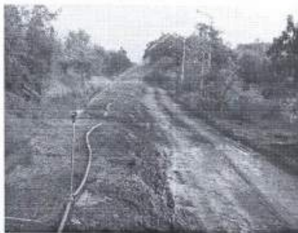
Continuous water sprinkling system for dust suppression
