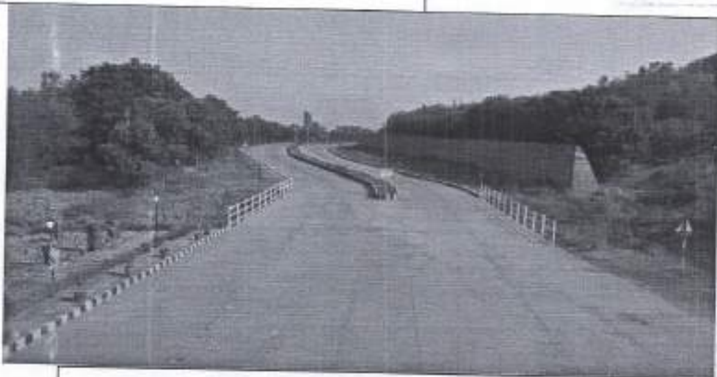
C.C.Road used as main haul road
