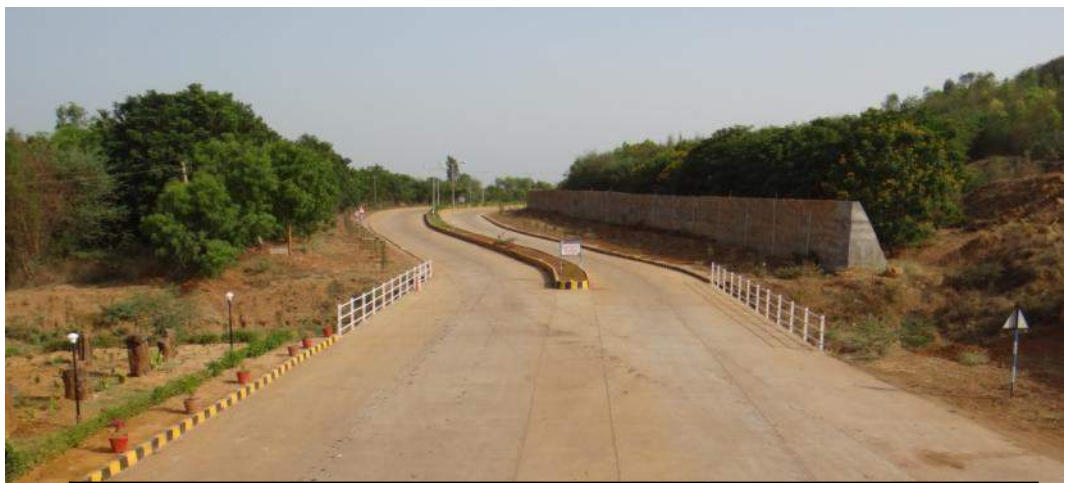
C.C.Road used as main haul road
