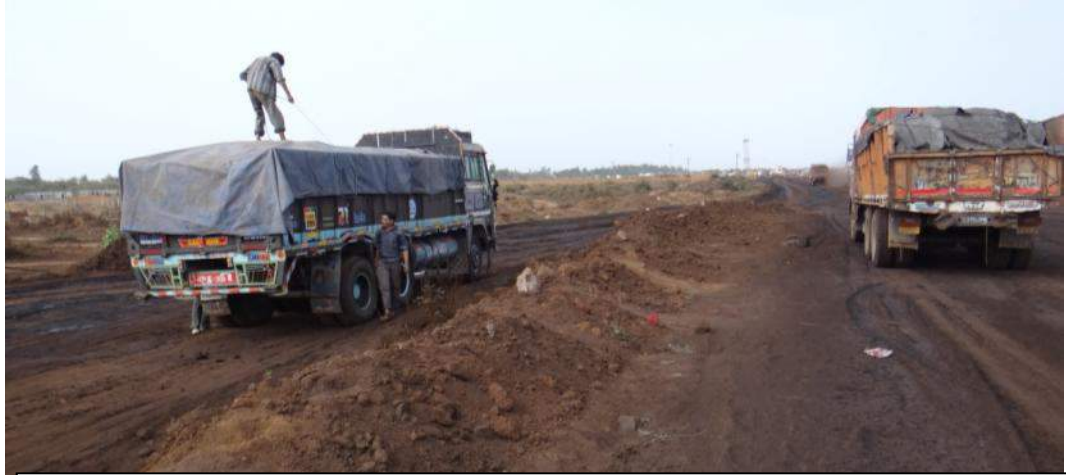
Covering with Tarpaulin of Loaded Trucks
